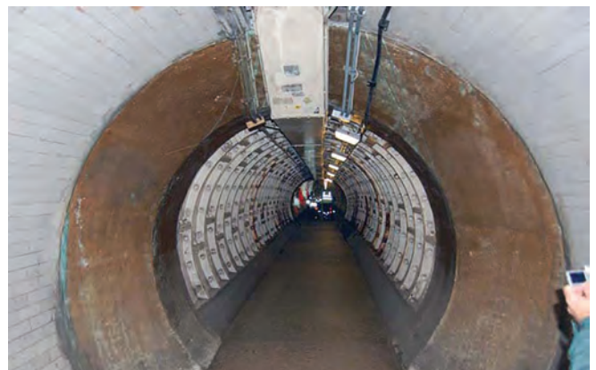
Repaired section of Greenwich foot tunnel, following damage in WWII
